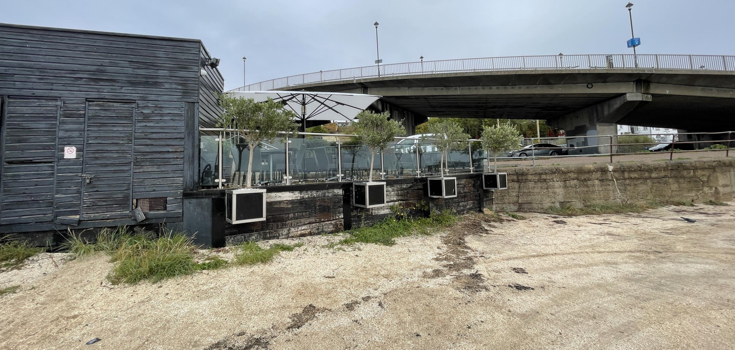
South Elevation showing Existing External Terrace and Existing Doors to Storage Area
